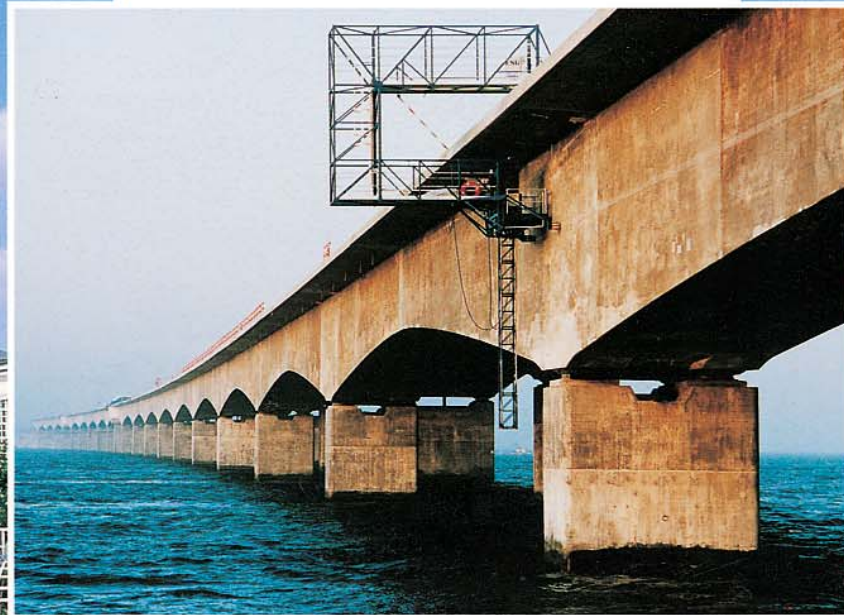
Storebaelt west bridge (DK)
